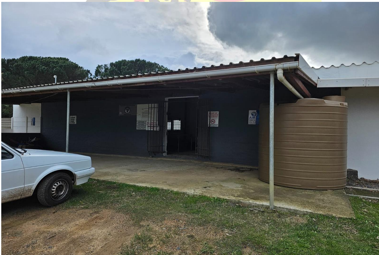
Figure 4.) Structures on site current- Clubhouse and main range (actual)
