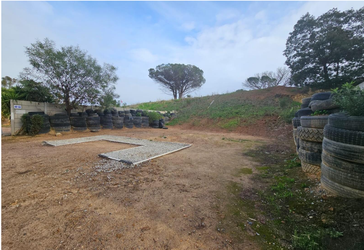
Figure 5.) Structures on site current- tyre wall (actual)
